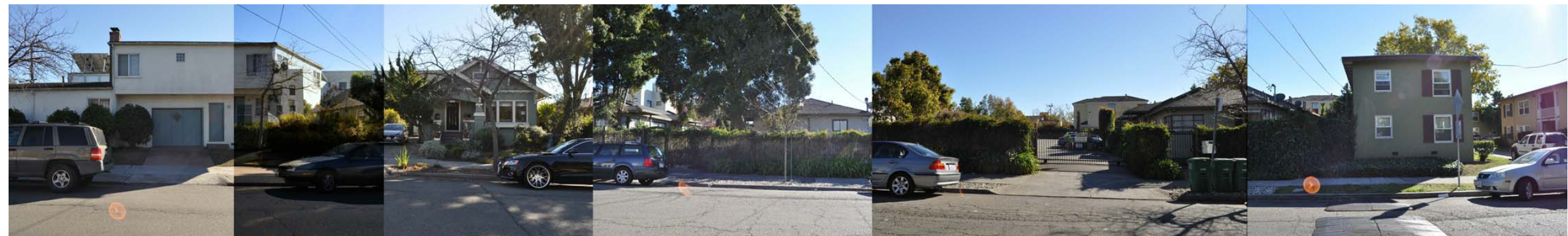
Existing Hearst Ave Strip, South
